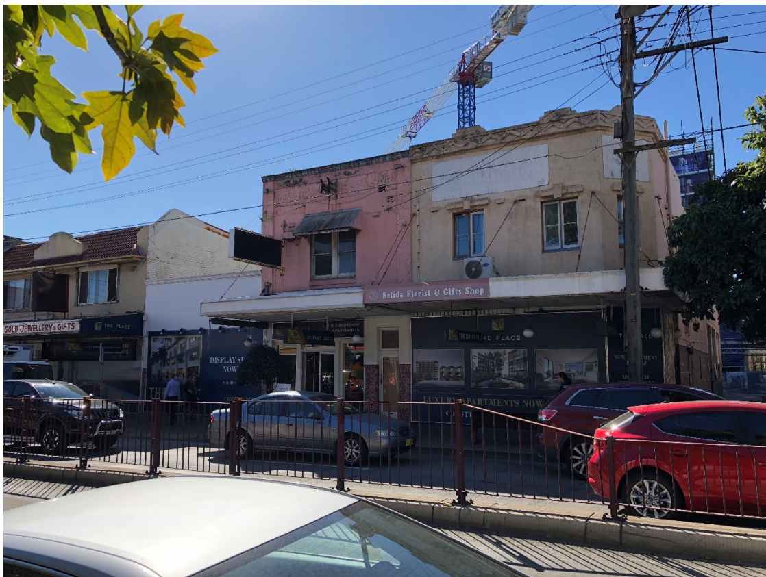
Picture 2 Site Photo – Ramsay Street frontage
